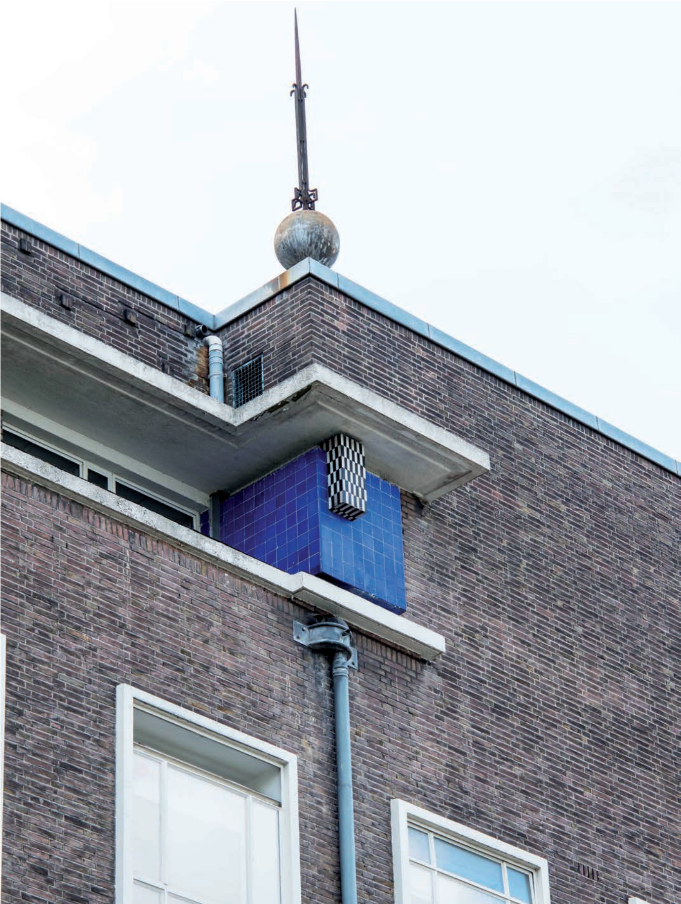
Facade decoration using coloured tiles.
