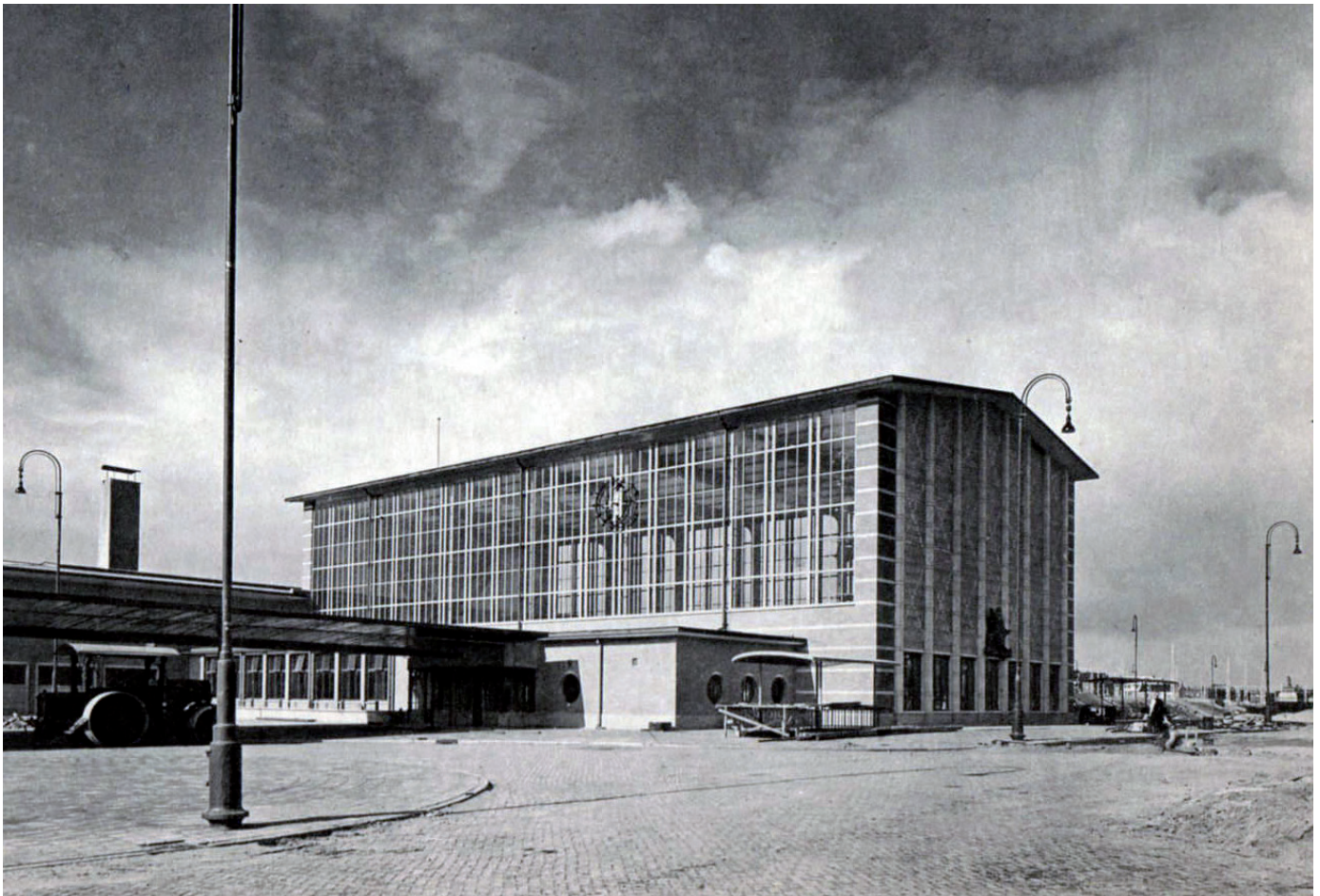
The original situation.
